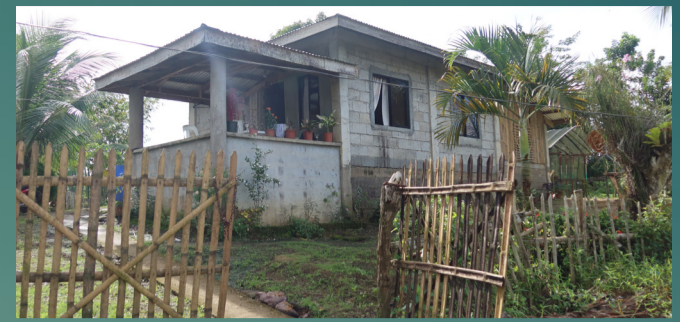
People would be surprised to see that Robelyn's home is made of concrete, instead of just light materials. She explains that having a solid house is necessary for the people of Cogon.
